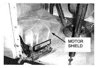
Disconnect the wires to the original motor.
